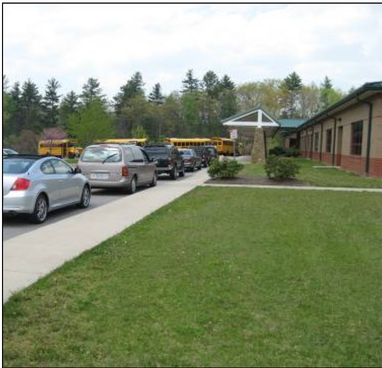
Photograph 8 – Student drop-off area in front of Greenlee School with opportunities for bioretention, downspout disconnection and rainwater cistern retrofit.
