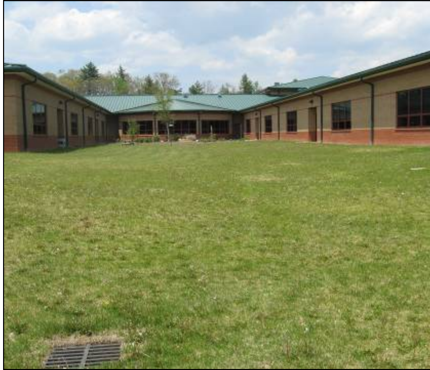
Photograph 3 – Courtyard at Greenlee School with opportunity for LID BMP retrofit.
